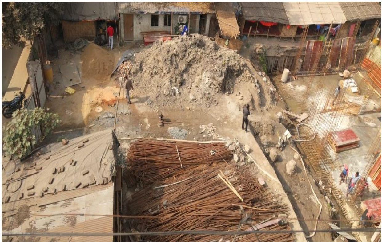
Stitching Slab and Retaining Wall Casting
